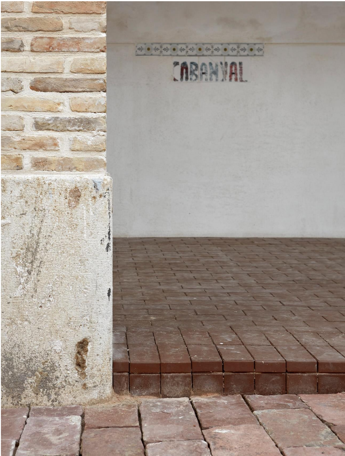
Current interior detail of the building. Source: https://www.fotografadearquitectura.com/wp-content/uploads/2022/05/Escorxador_36.jpg
